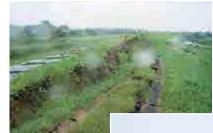
Bund breaking by North Miyagi earthquake (Naruse River, Miyagi pref.)
