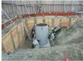
Photo 5 - Installation status of ring socket
